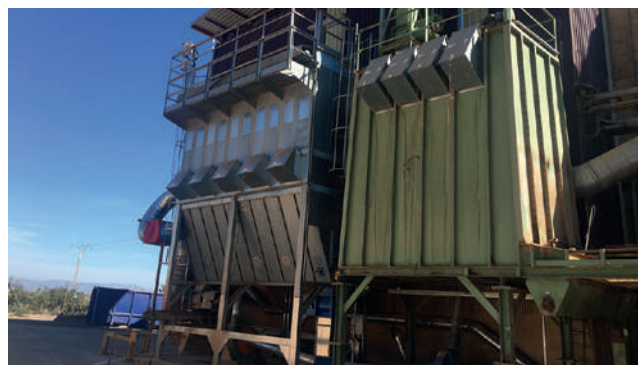
Figura 13. Interior de silos, tolvas, etc.
